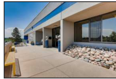
JLL provided acquisition funds for 7070 S. Tucson Way in Centennial.
